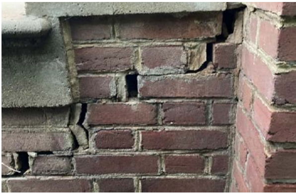
1" of forward movement has occurred at top step.
